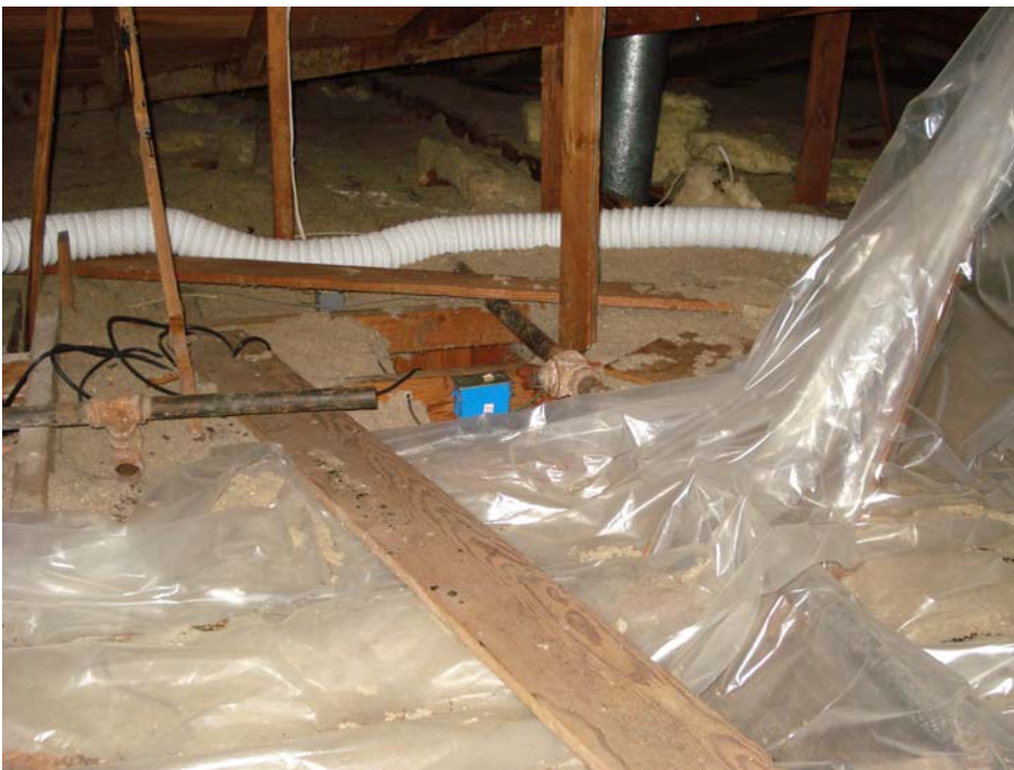
Return Duct in Attic
