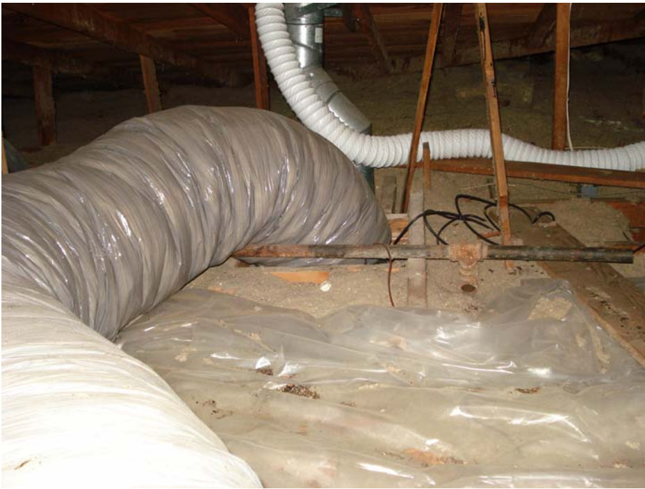
Return Duct in Attic
